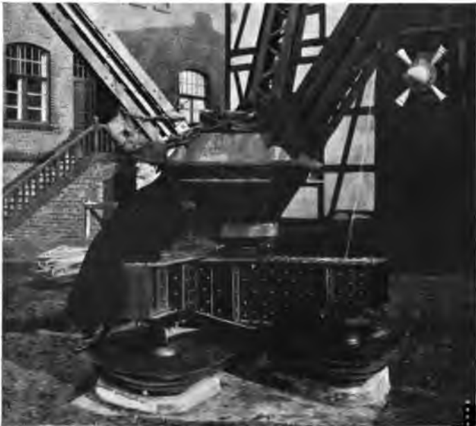
FIG. 135.—Foot of aerial tower showing insulation from ground. [See p. 275.]
